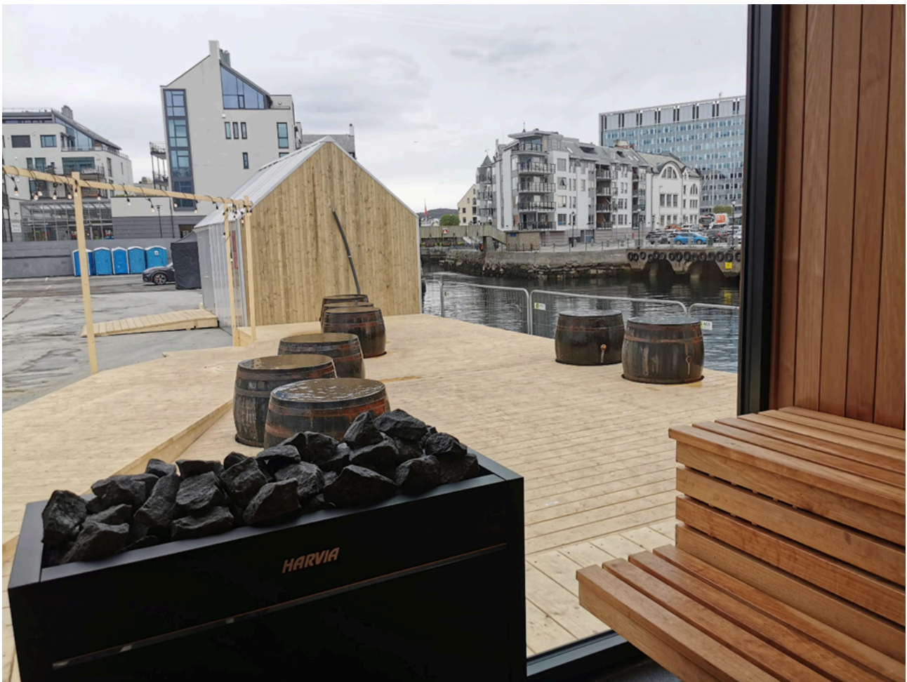
Temporary sauna on the site of the future Kulturhavna and the previous bathhouse (Photo: SUAS)
