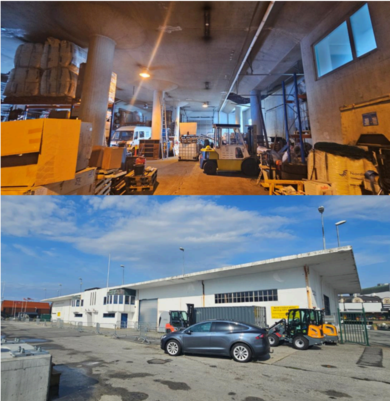
Devold building before renovation (photo: ÅK)
