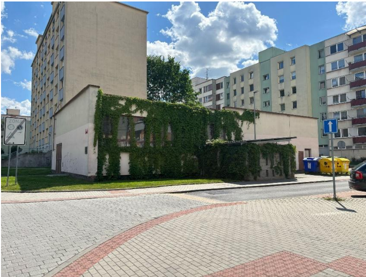
Figure 14: Photo of the heat exchanger station at Partyč housing estate, May 2025, photo by Jan Roucka
