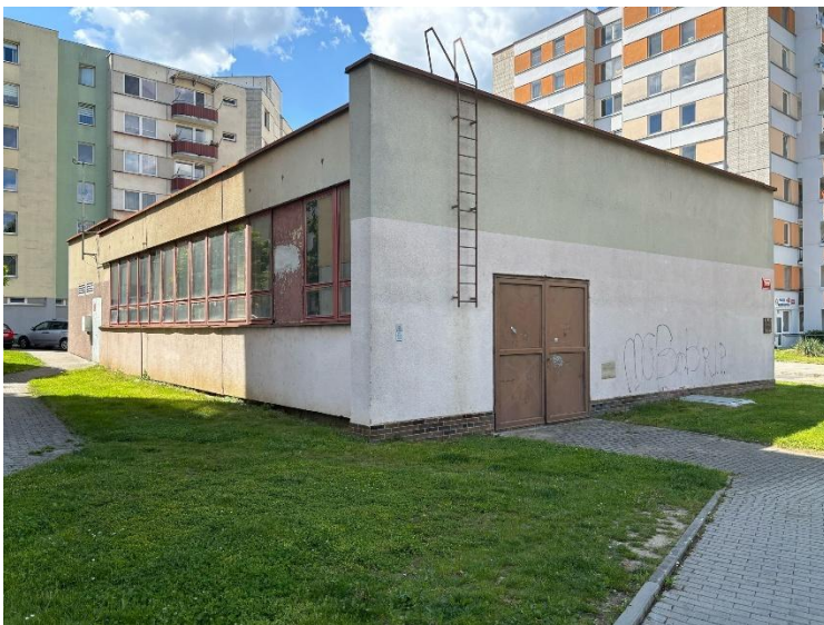
Figure 13: Photo of the heat exchanger station at Portyč housing estate, May 2025, photo by Jan Roucka
