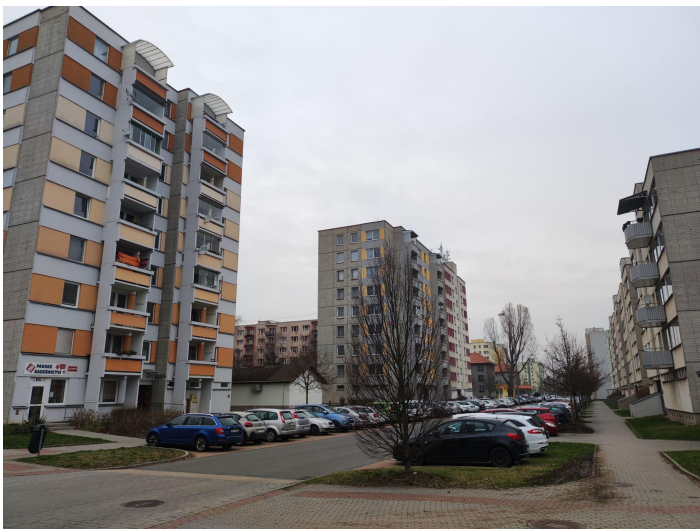
Figure 2-3: Photos of the Portyč housing estate 2024, photo by Jan Roucka
