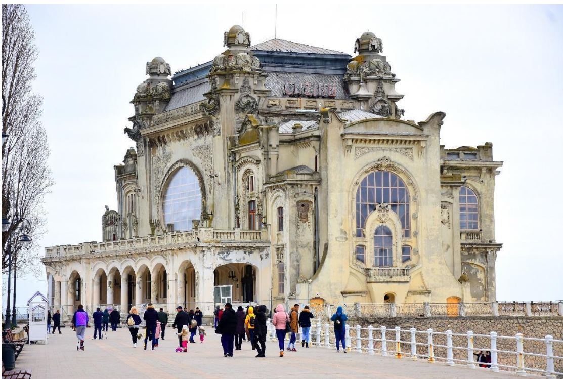
Fig. no. 27: Constanța Casino building before refurbishment (source: Constanța municipality)
