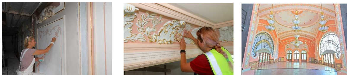
Fig. no.28: Casino building refurbishment process and outcomes (source: Constanța municipality)
