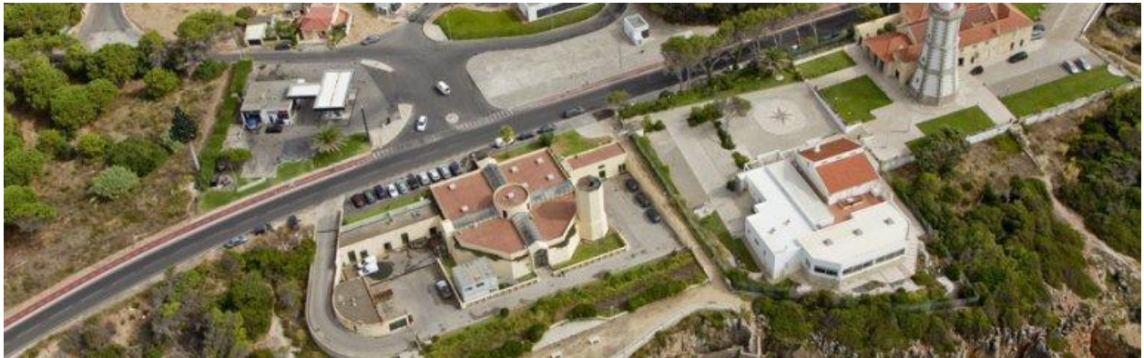
Figure 7: Guia Wastewater Treatment Plant – Liquid Phase 3 .
