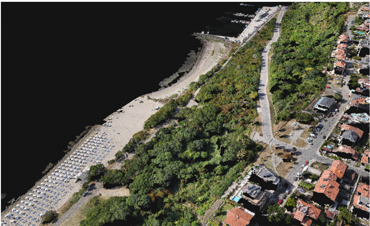
Fig. 22. Angled visualization of a 3D point cloud obtained from an aerial photogrammetric survey of the Project Territory - western part
