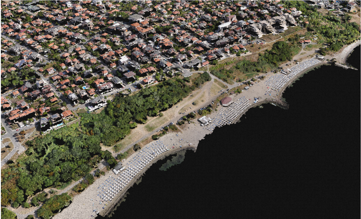
Fig. 23. Angled visualization of a 3D point cloud obtained from an aerial photogrammetric survey of the Project Territory – middle part, Source: Sofia University “Saint Kliment Ohridski”
